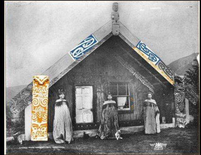
Giles Quarme & Associates Dimensions of Hinemihi 05-06-00 scaled perspective photograph, Burton Brothers; agreed width - 6.7m agreed height - 3.9m suggested length - 12.7m
