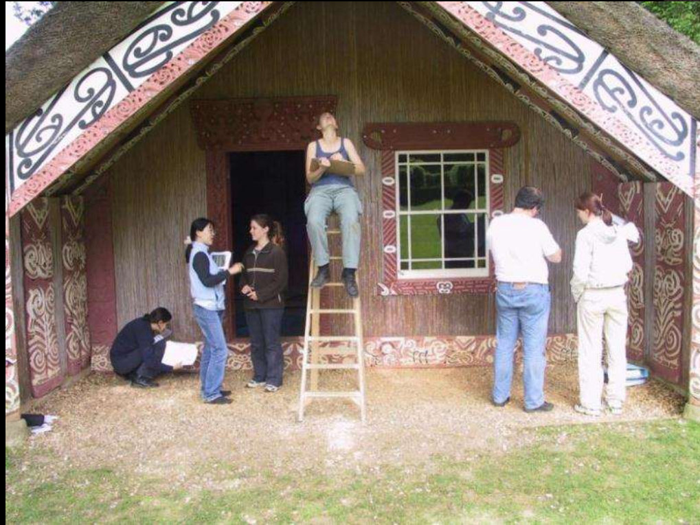
UCL conservation students conducting a condition survey of Hinemihi, 2003
